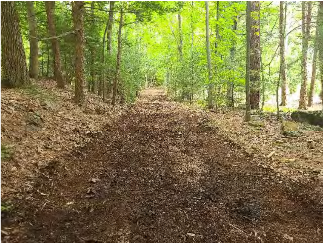
Fig 26: Restoring access road off Foss Farm Rd. Viewing southwest. (07-22-20).
