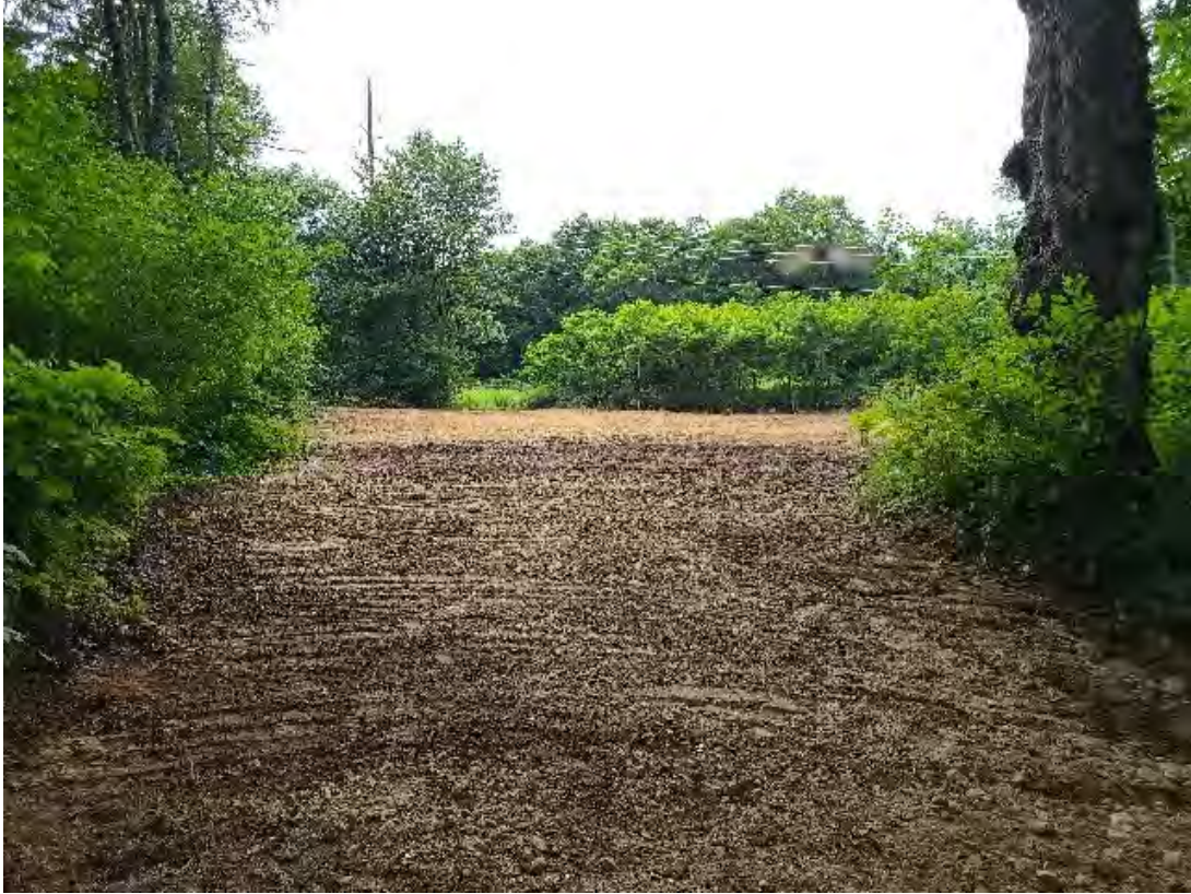
Fig 27: Restoring staging area off Foss Farm Rd. Viewing southwest. (07-22-20).
