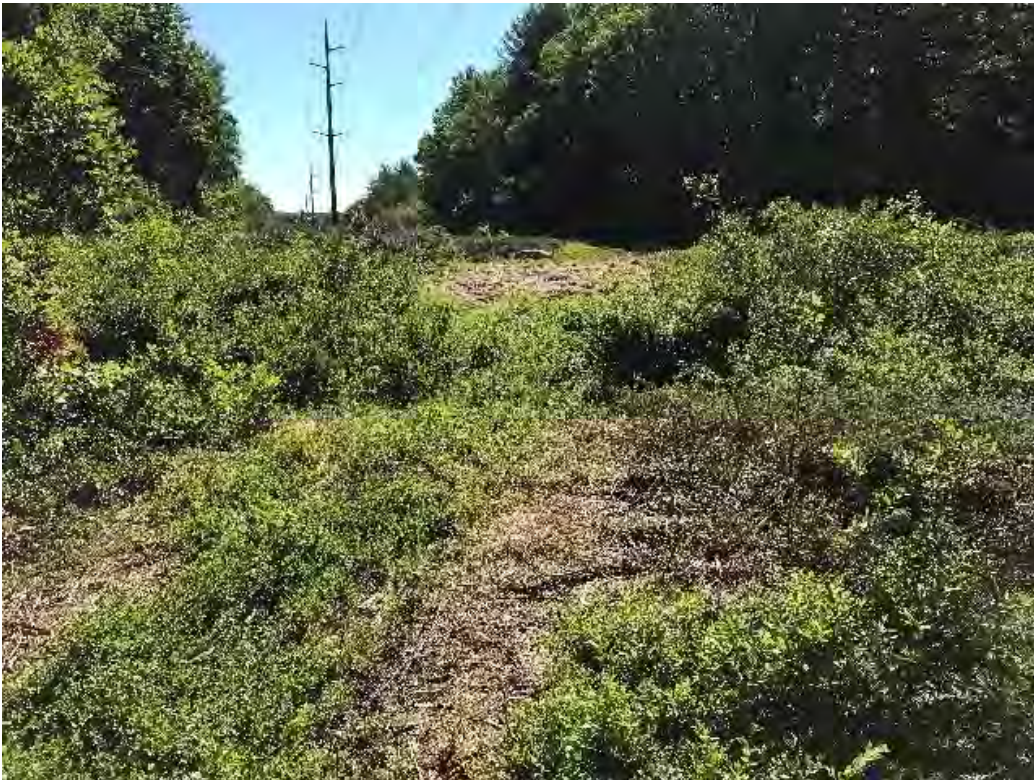
Fig 14: Re-vegetating access road crossing of wetland DW40. Viewing east. (07-21-20).
