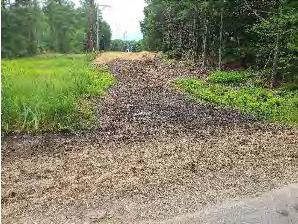
Fig 23: Wetland DW12 off Durham Point Rd. restored. Viewing southeast. (07-22-20).
