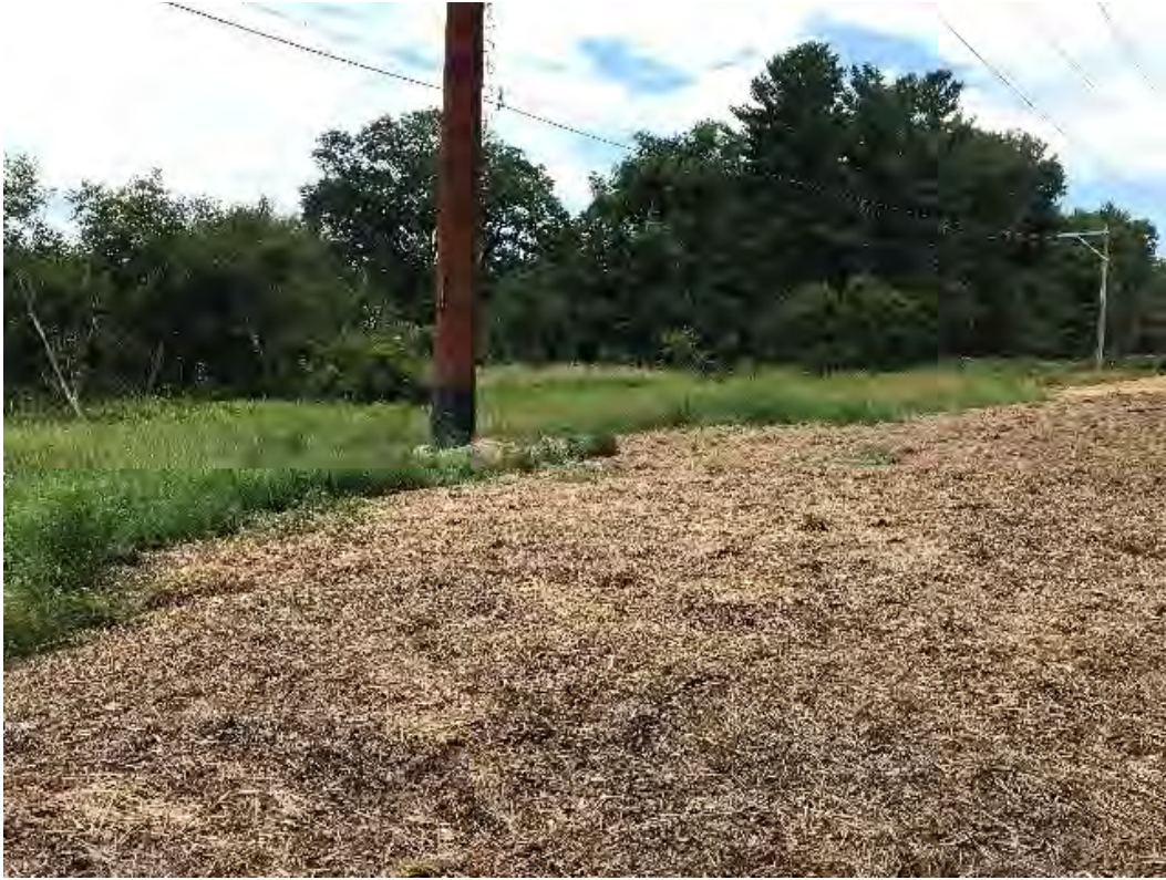
Fig 11: Str. 95 work area restored. Viewing west. (07-20-20).
