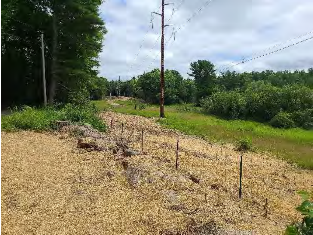
Fig 3: Access route between Strs. 94 and 95 restored. Note replacement fence. Viewing southeast. (07-16-20).
