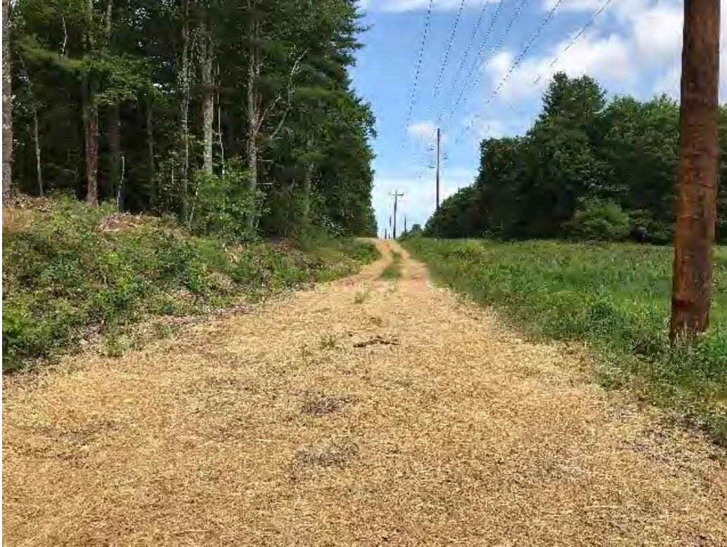
Fig 13: Access road between Strs. 93 and 92 restored. Viewing northwest. (07-20-20).
