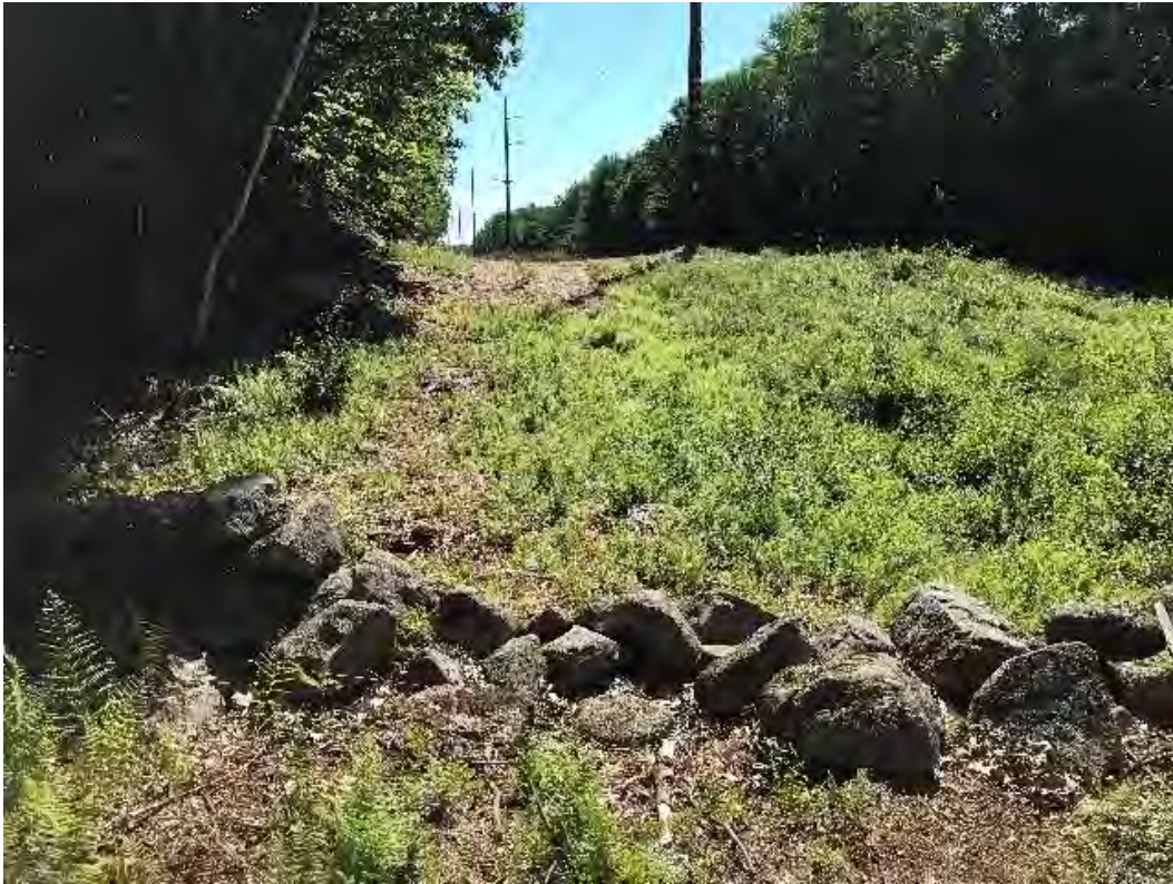
Fig 15: Re-vegetating access road with stonewall adjacent to wetland DW27. Viewing east. (07-21-20).
