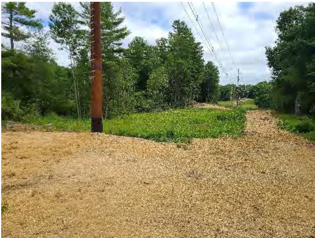
Fig 2: Str. 94 work area restored. Viewing northeast. (07-16-20).
