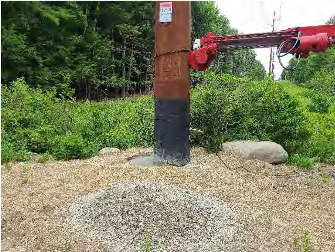
Fig 25: Pouring float fill for Str. 70 foundation. Viewing east. (07-22-20).
